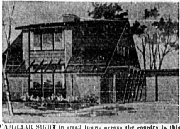
A FAMILIAR SIGHT in small towns across the country is this trim and proper little house constructed in the 1920's. Built solidly enough it is however out-dated, formal and unattractive with the old fashioned porch shutting out light and air. Its owners, like thousands of others, would like to modernize it—inside and out. Remodeling ideas for the 1923 home call for a modern "face-lift" of the drab exterior without basic structural change. Dark brick is faced with bright stucco, old front porch removed and living room extends out to new open eaves. Main entrance is moved to side of the house. A second side door replaces old back door, eliminating tracking in through front. New garage and sheltered walk are added. And, big new windows let in more light and air and add to modern appearance.
