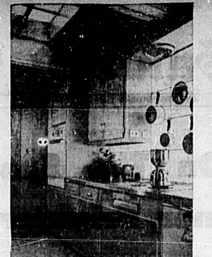
CONTROLLED DAYLIGHT ILLUMINATION is provided for this kitchen by two sources: a prefabricated top-lighting panel set in the roof and a vertical wall of prismatic glass block. Brightness ratios on sunny days are no brighter than they are on cloudy days, giving a daylight look always.
