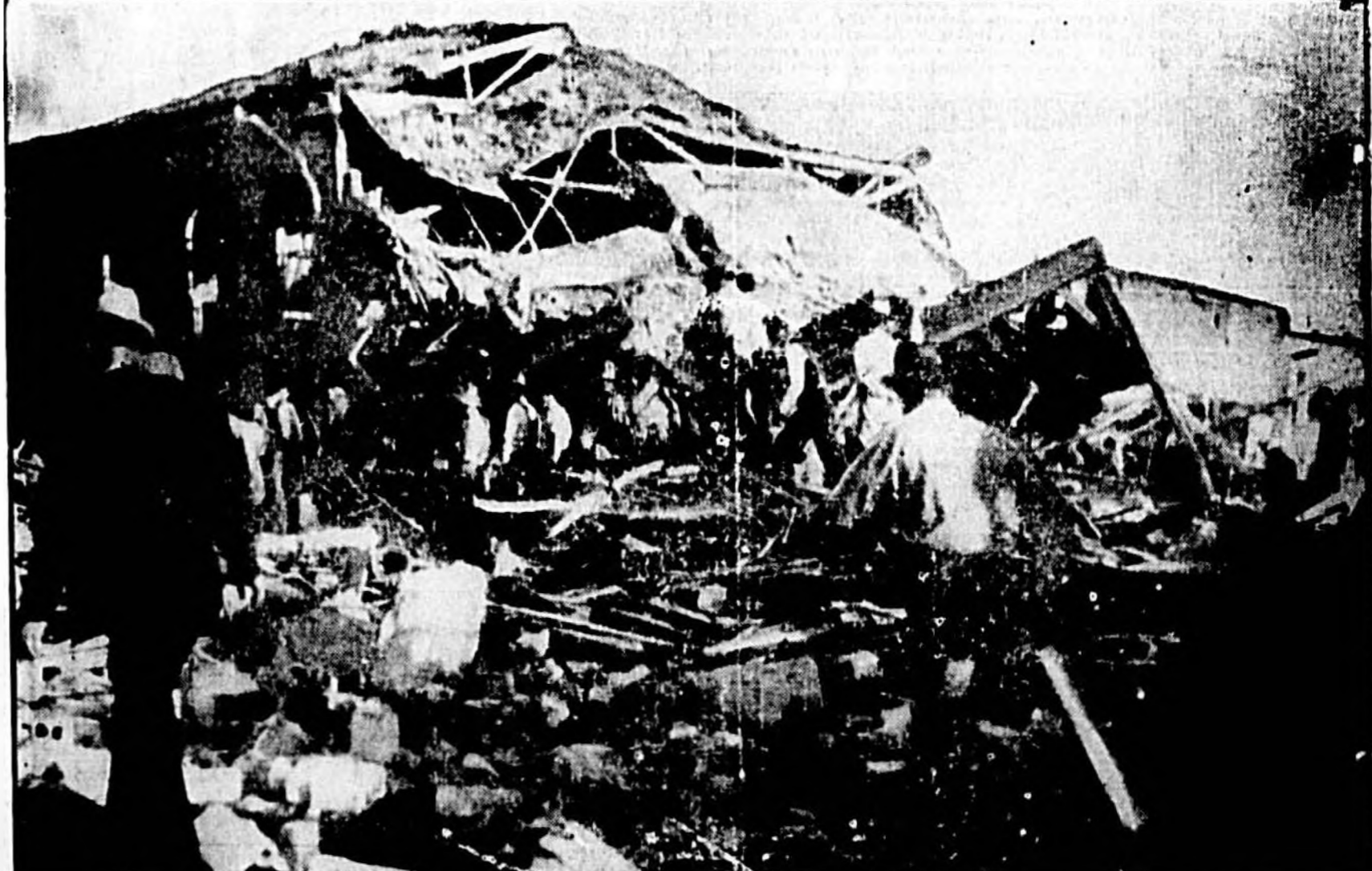
Somewhere beneath this ghastly pile of debris, hundreds of bodies lie buried as a consequence of an unexplained blast that wrecked the Consolidated school at New London, Texas. An army of rescue workers is shown digging into the mass in search of the dead. The quick recovery of 500 bodies gave rise to estimates that 670 were killed by the explosion. (Associated Press Photo)
