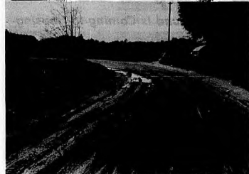
Unpaved roads like Vihlen Road west of Sanford are located throughout Seminole County and are expensive to maintain because they wash out
