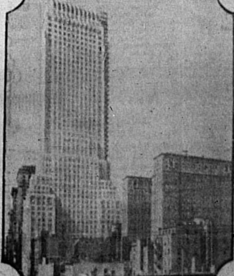
New York's new structural pride is the Chanin Building, now nearing completion, on 4th Street at Lexington Avenue and opposite the Grand Central Terminal. The structure is 600 feet high, or about a hundred feet shorter than the Woolworth Building.
