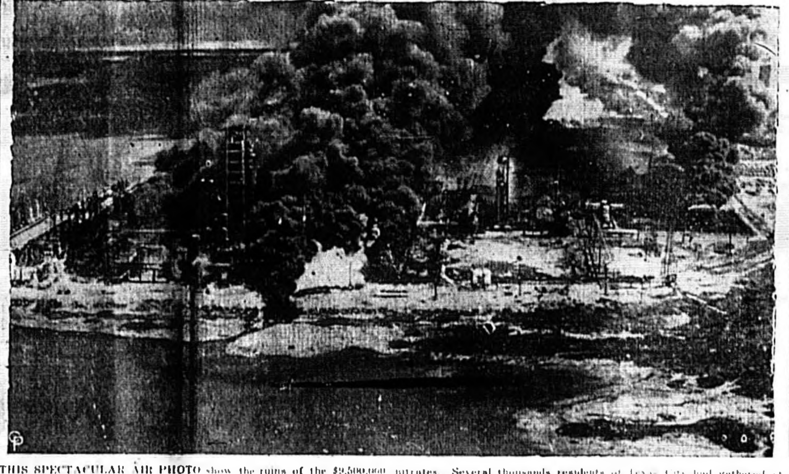
THIS SPECTACULAR AIR PHOTO shows the ruins of the $9,500,000 Monsanto Chemical Plant in Texas City, Tex., which was destroyed in the explosion and fire that virtually razed Texas City, Tex., and brought a death toll estimated at more than 1,000 persons.
