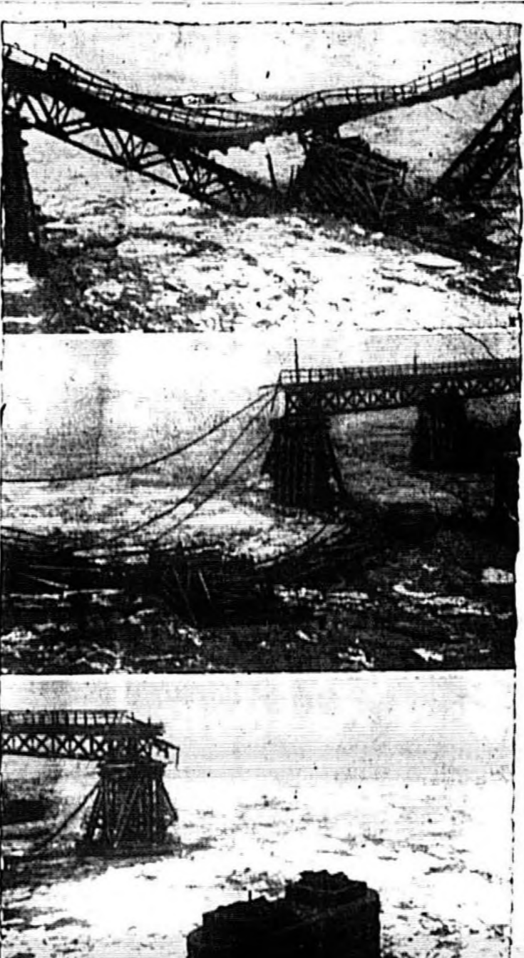
A TEMPORARY SPAN crossing the Vistula River in Warsaw, Poland, is pictured by News of the Day Newsreel as heavy flows of river ice buffeted against the wooden-piling supporting the main span, causing the bridge to collapse. The bridge starts to give way (top) then drops into the roaring torrent (center) and is completely swept away (bottom) by the unleashed fury of the floodwaters.
