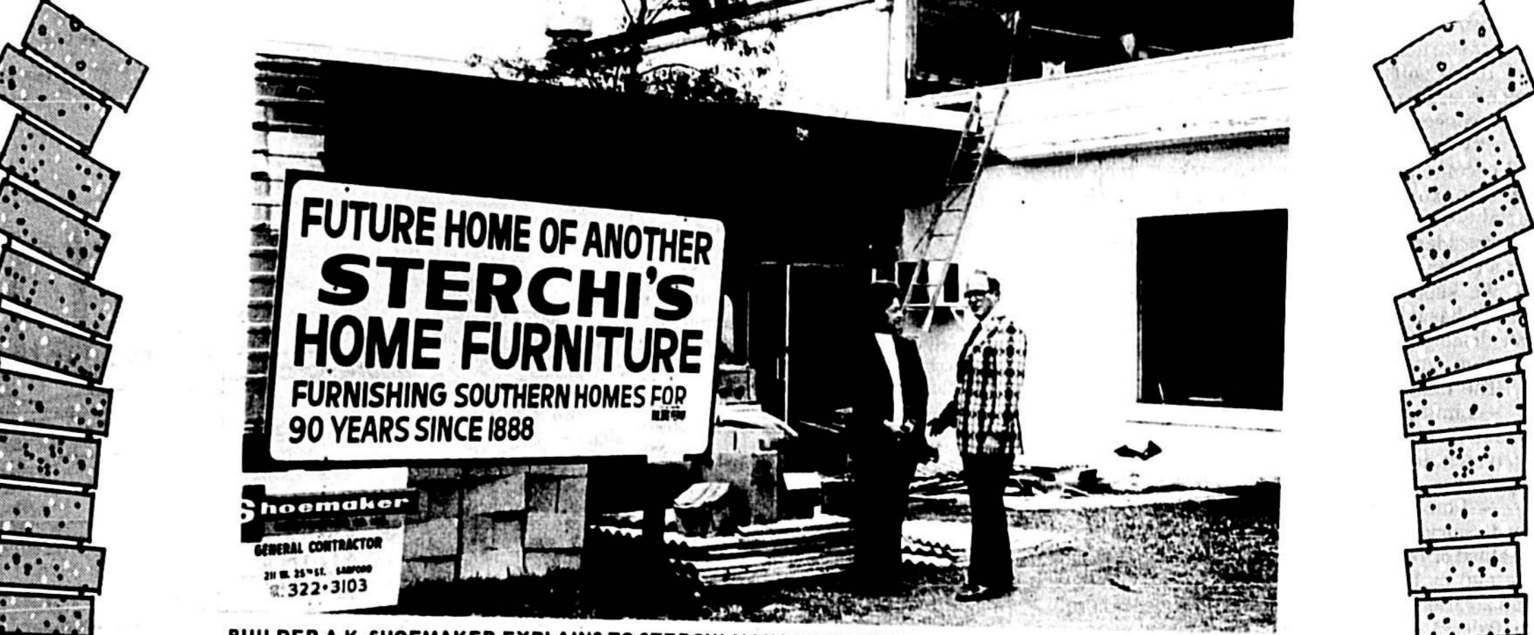
BUILDER A.K. SHOEMAKER EXPLAINS TO STERCHI MANAGER FAYE ROBERTS THAT MERCHANDISE MUST BE MOVED TO MAKE ROOM FOR EXPANSION AND REMODELING NOW IN PROGRESS.
