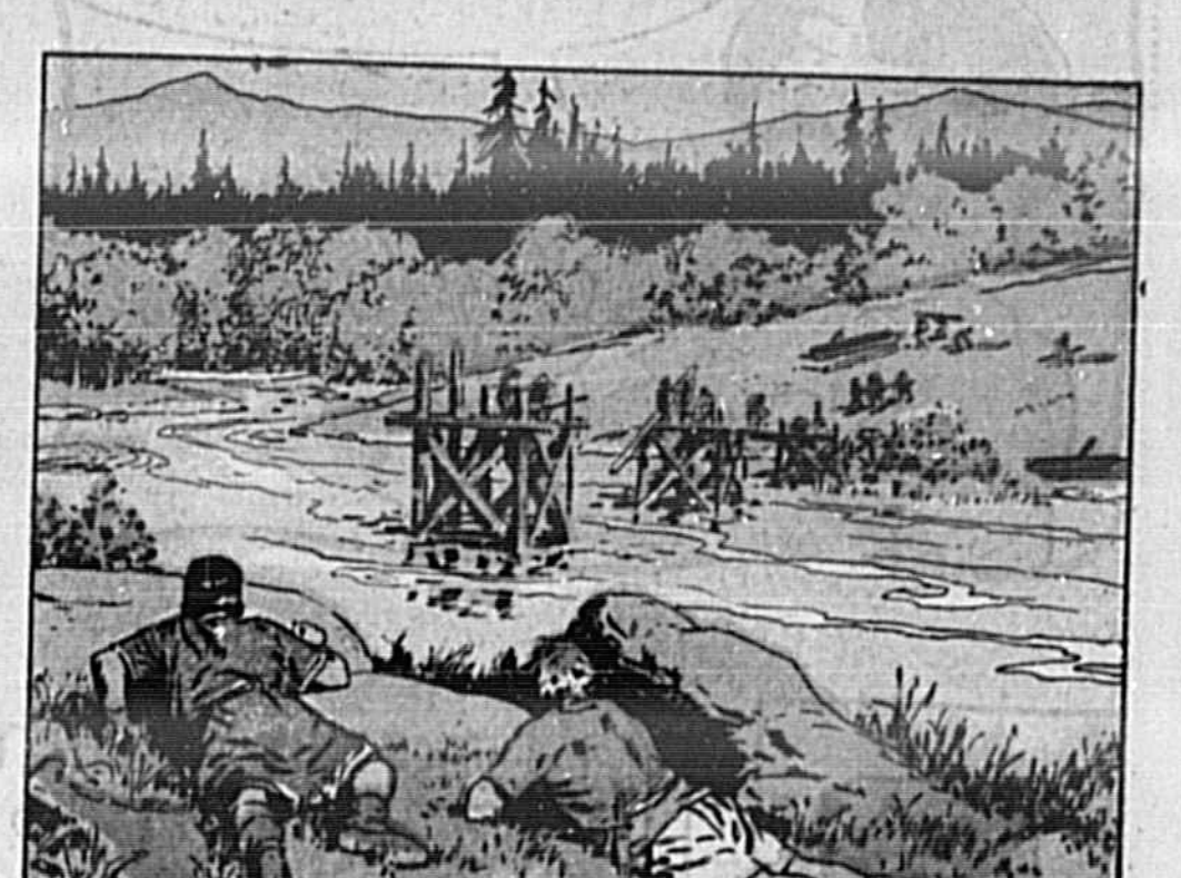
WHERE THE RIVER WIDENS AND FLOWS GENTLY OVER A GRAVEL BED, A BRIDGE IS UNDER CONSTRUCTION. UNTIL IT IS FINISHED, THE INNER LANDS WILL BE SAFE FROM INVASION.
