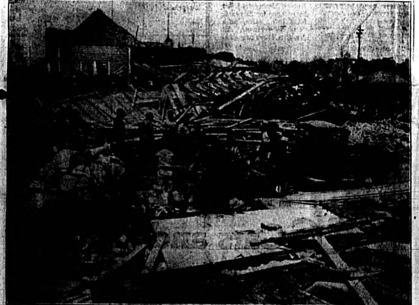
Hundreds of demolished houses were left in Cordele, Ga., in the wake of a tornado that dipped twice, killing 14 persons, injuring thousands more and doing damage estimated at $1,000,000. This picture shows a general view of the debris in one of the residential districts. (AP Photo)
