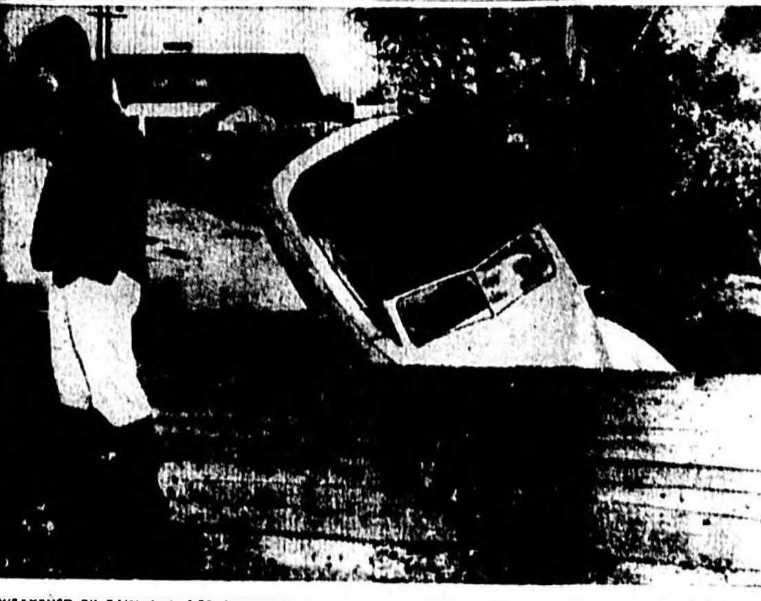
WEAKENED BY RAIN AND FIERCE WINDS, the approach to this bridge in Squilam, Washington, gave way and trapped a passing automobile. At least 100 of the worst storms in Pacific Northwest history, Washington, Oregon and British Columbia were threatened with major destruction as rain-soaked streams threatened to break over banks. Thousands of acres of land were inundated.
