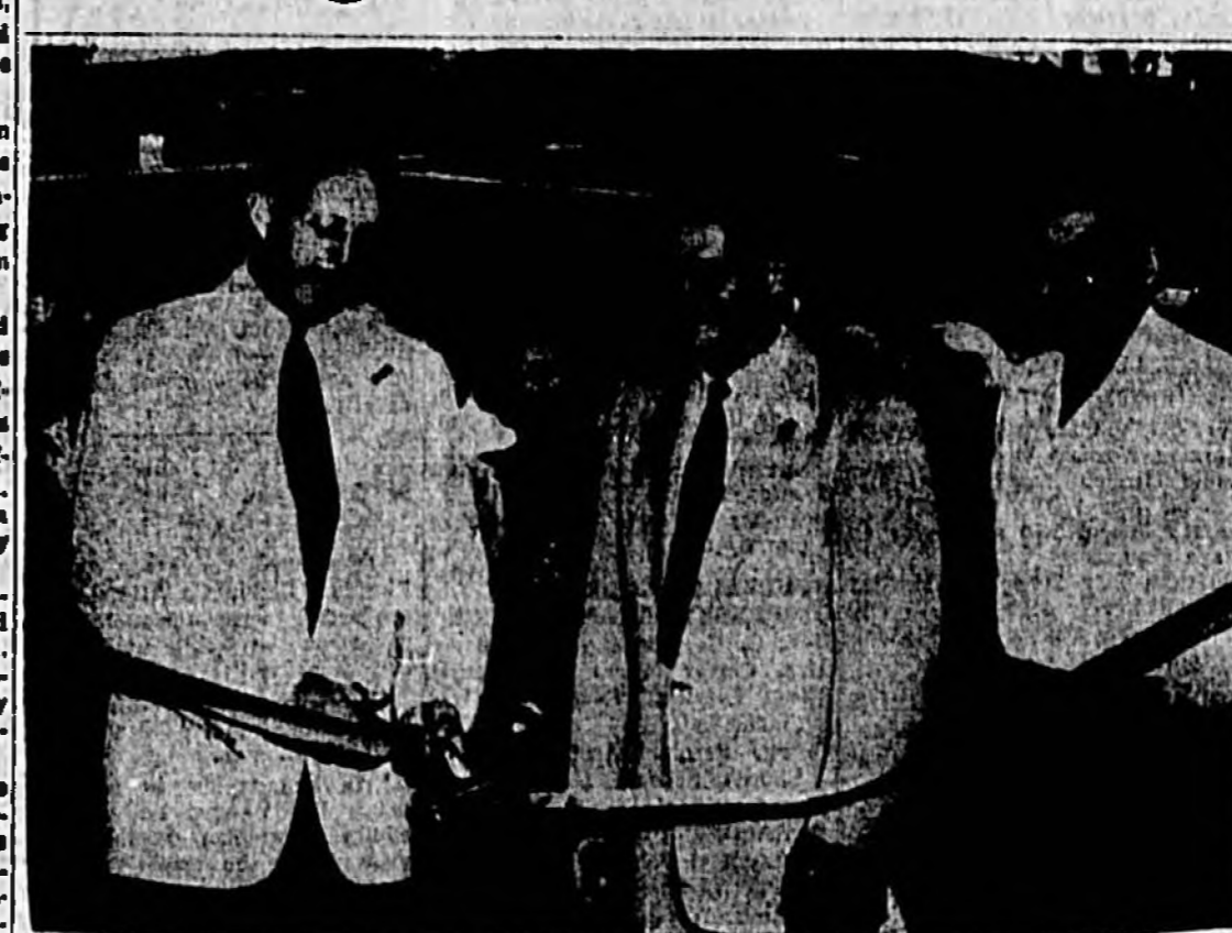
MAYOR F. D. SCOTT OFFICIALLY opens the brand new $25,000 Therm-O-Tane Gas and Appliance Co. building this morning when he cut the ribbon to allow a huge crowd already waiting to visit the ultra-modern show rooms, offices and warehouse located on the corner of West 9th St. and Laurel Ave. With Mayor Scott is C. H. Robertson, vice president of the company. (Staff Photo)
