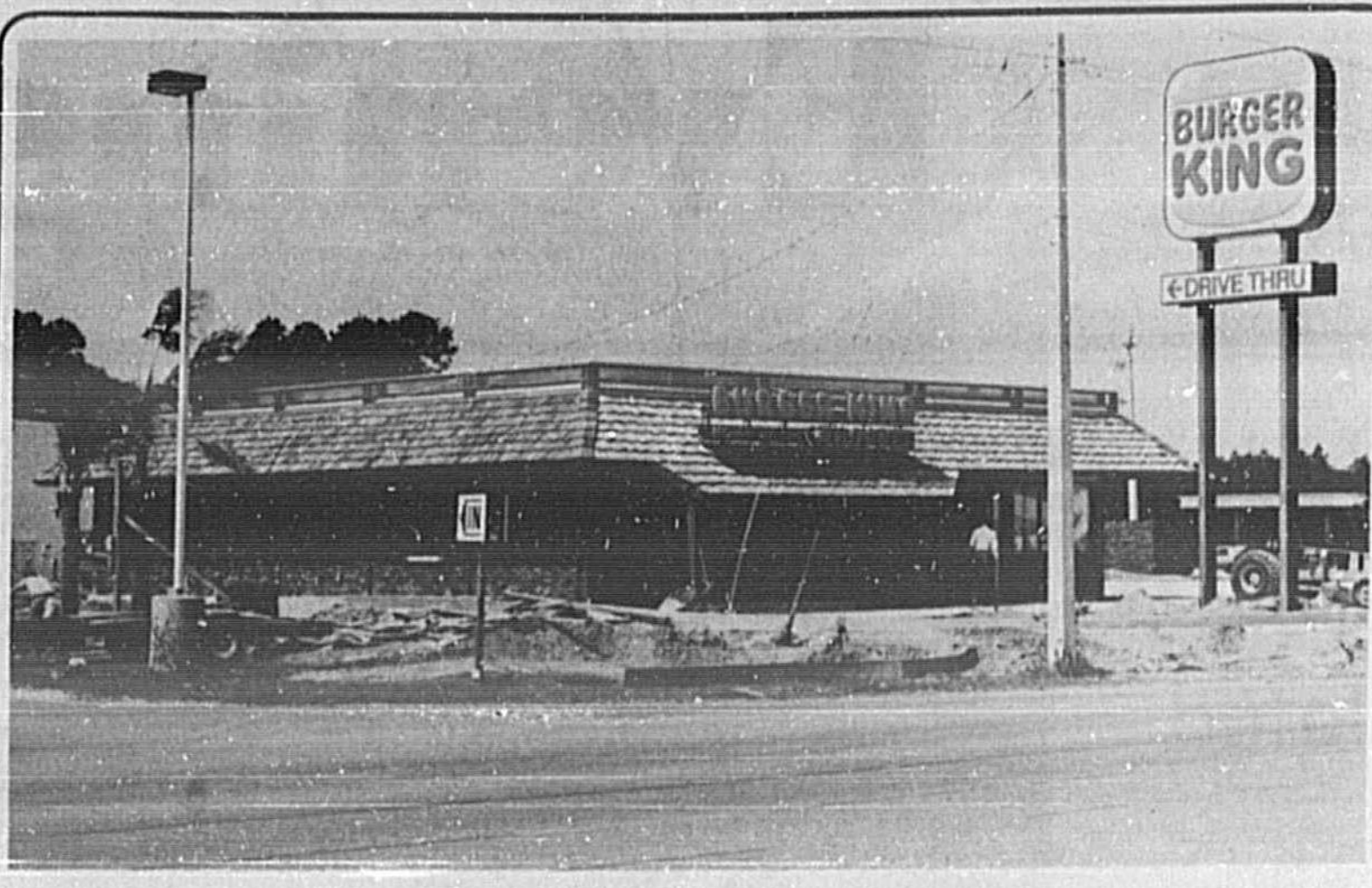
EATING PLACES NEAR COMPLETION
