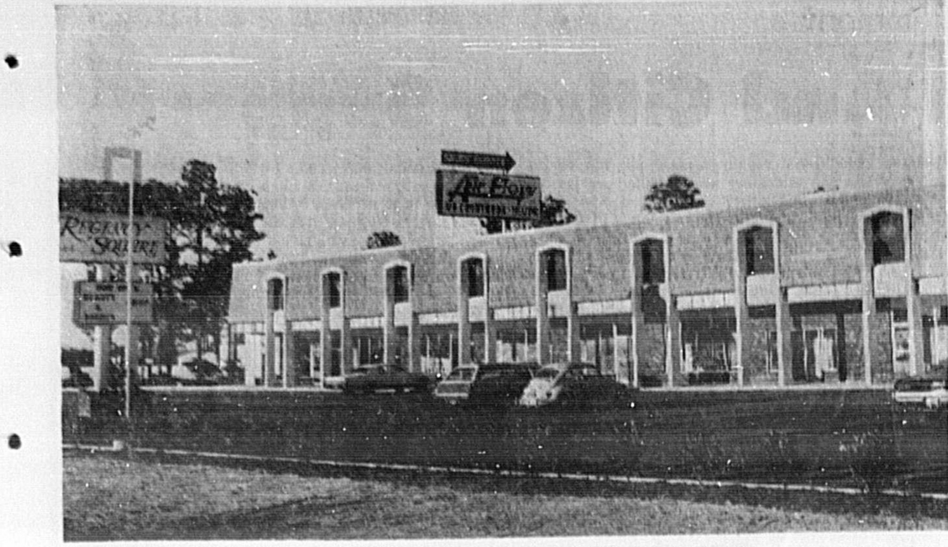
REGENCY SQUARE on SR 436, Casselberry, a business and professional center built at the cost of $250,000 by R. O. Cousineau of Casselberry, owner, is readying the various shops and restaurants for opening around the first of the year. A barber shop and beauty parlor are already open and opening in the near future will be a laundry, dry cleaner, dress shop, a western restaurant, piano and organ dealer, and Sanderette. The professional suites on the second floor will be served by the city's first elevator. (Jane Casselberry Photo)
