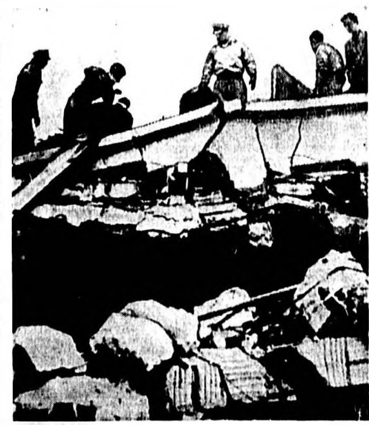
SOLDIERS AND CIVILIAN VOLUNTEERS probe the wreckage of a building after an explosion rocked the downtown section of Guatemala City, Guatemala. Fifty persons were killed by the force of the blast and by falling walls. An entire block was almost destroyed. (International)
