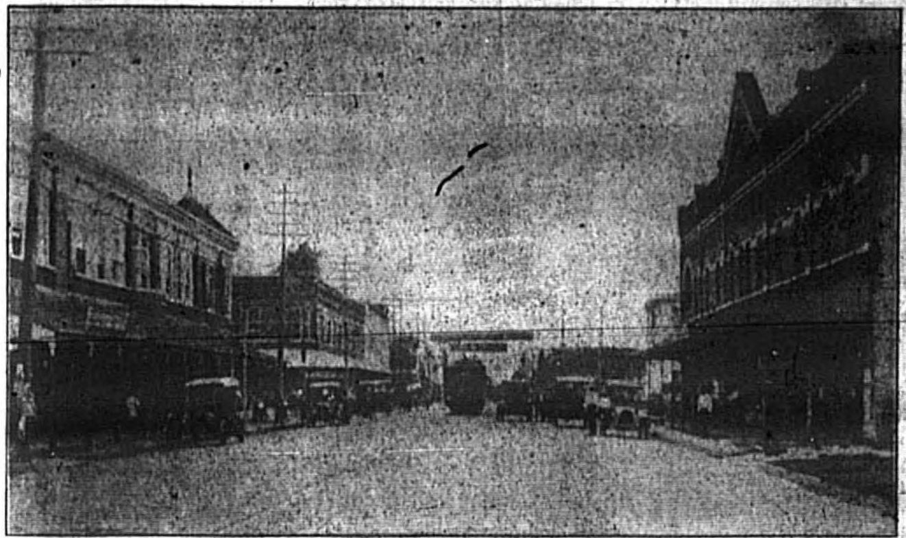
LOOKING WEST ON FIRST STREET
