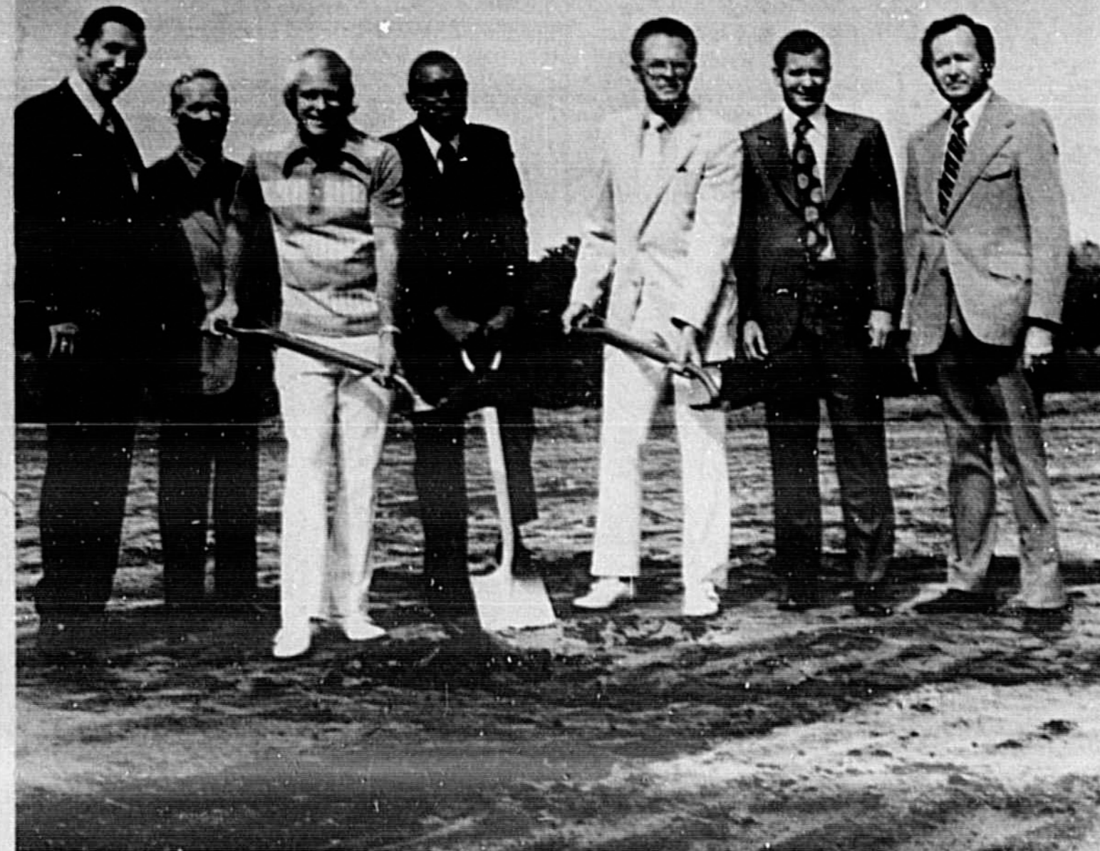
GROUND-BREAKING for new Concrete Structural Systems Inc. plant at Port of Sanford was held Friday morning on the site of the new firm, which is expected to employ about 100 persons, when completed. Attending the festivities were members of the Seminole County Port Authority (SCOPA) Citizens National Bank of Orlando, Concrete Structural Systems and Seminole County Rep. Gene
