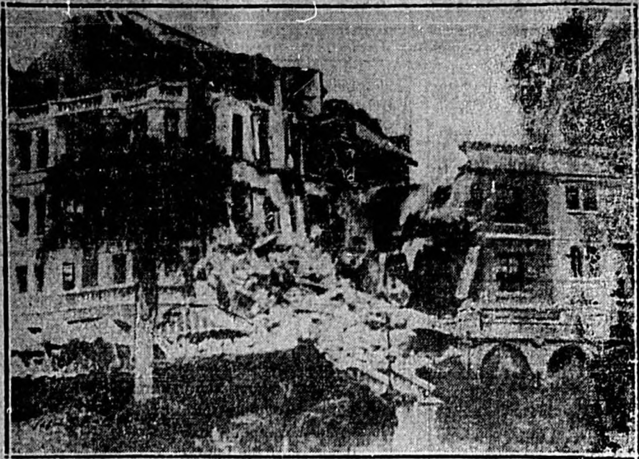
Several persons sleeping in the Arlington Hotel at Santa Barbara were killed when the earthquake tore a great gap in the structure and sent rooms on the third floor crashing to the street below. The ruins of the hotel are strikingly shown in the photograph above. The wreckage, under which the victims were buried, is piled in the street.
