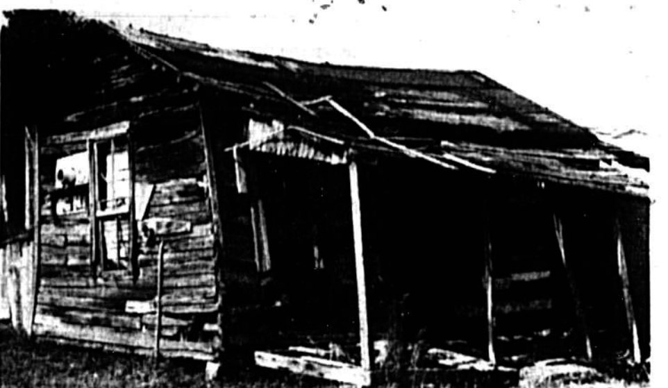
Seminole County will use its new condemnation ordinance to rid the county of unoccupied, hazardous structures such as this abandoned building in the Bookertown area west of Lake Monroe, according to county building official Don Flippin.
