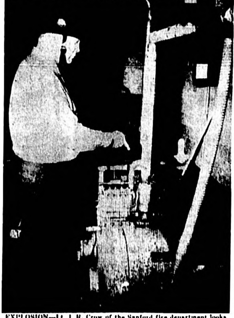
EXPLOSION—Lt. J. R. Crow of the Sanford fire department looks at a broken connection (arrow) in the air conditioning system at Lovell's, Third St. and Palmetto, where an explosion occurred yesterday. A wall dividing the motor room and the men's room was blown loose and the door of the latter room was blown off. No one was in either room when the explosion occurred. (Staff Photo)
