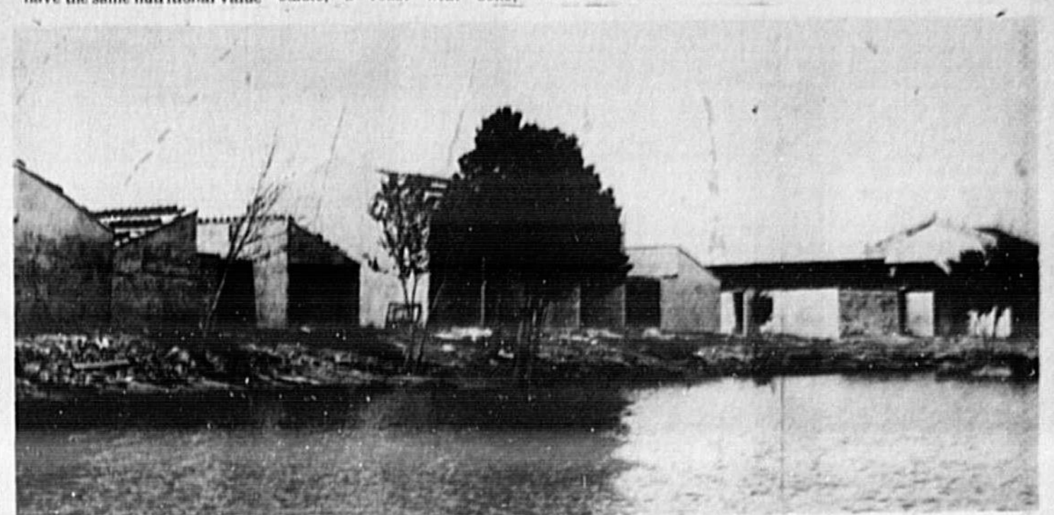
SAUSALITO UNDER CONSTRUCTION
