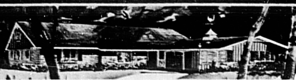
EARLY AMERICAN-STYLE RANCH is designed for the growing family. Built-in house two more bedrooms and a full bath. The room is an imaginative and sensible home in itself, also. There is a dramatic sunken living room with fireplace and beamed ceiling. The dining room, kitchen and dinette are well located, with the laundry nearby. There also is a laundry and mudroom, an attached garage and an abundance of closets. Plan HAT23 contains 1,206 square feet and was designed by architect Samuel Paul, 107-40 Queens Blvd., Forest Hills, N. Y. 11375, who may be written for further information.
