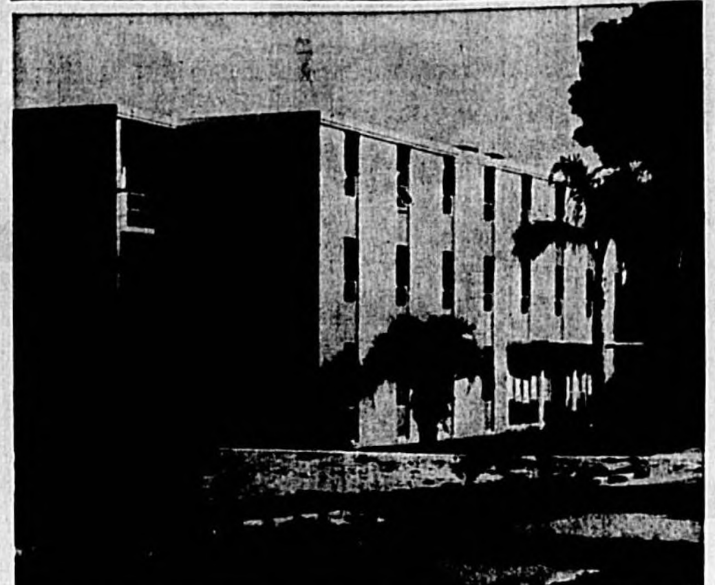
THE BRAND NEW GIRLS residence hall was recently completed on the Forest Lake Academy campus. It also was constructed by Groves Builders. Another wing on the dormitory is expected to start next week after school is out.
