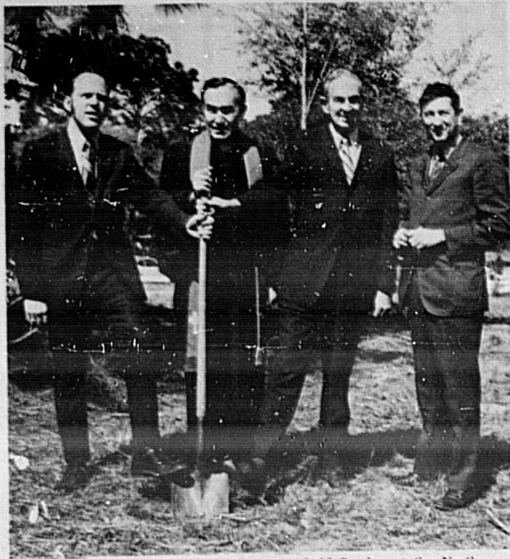
GROUND BREAKING ceremonies were held Sunday at the North Street site in Rolling Hills for St. Marks Presbyterian Church. Construction will begin immediately on the $214,000 structure. Left to right, Earl Eberly, chairman of building committee; Rev. Harvey Walters, pastor; Dean Larrick, planning committee chairman, and Tom Hunter, architect.
