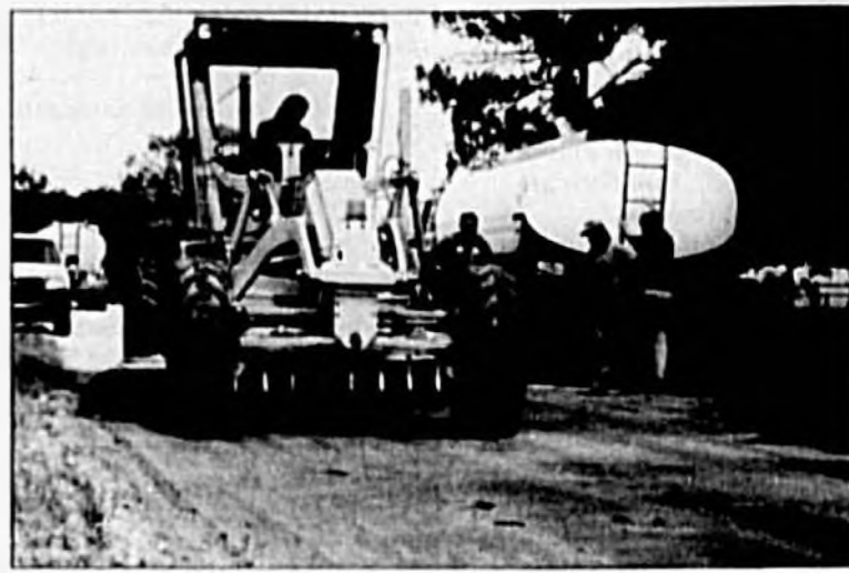
Photo submitted by Dave Heeselman Tad Wheeler of Zephyr Stripe and Seal and other members of the crew watch the application of Pennzsuppress D in Sanford.
