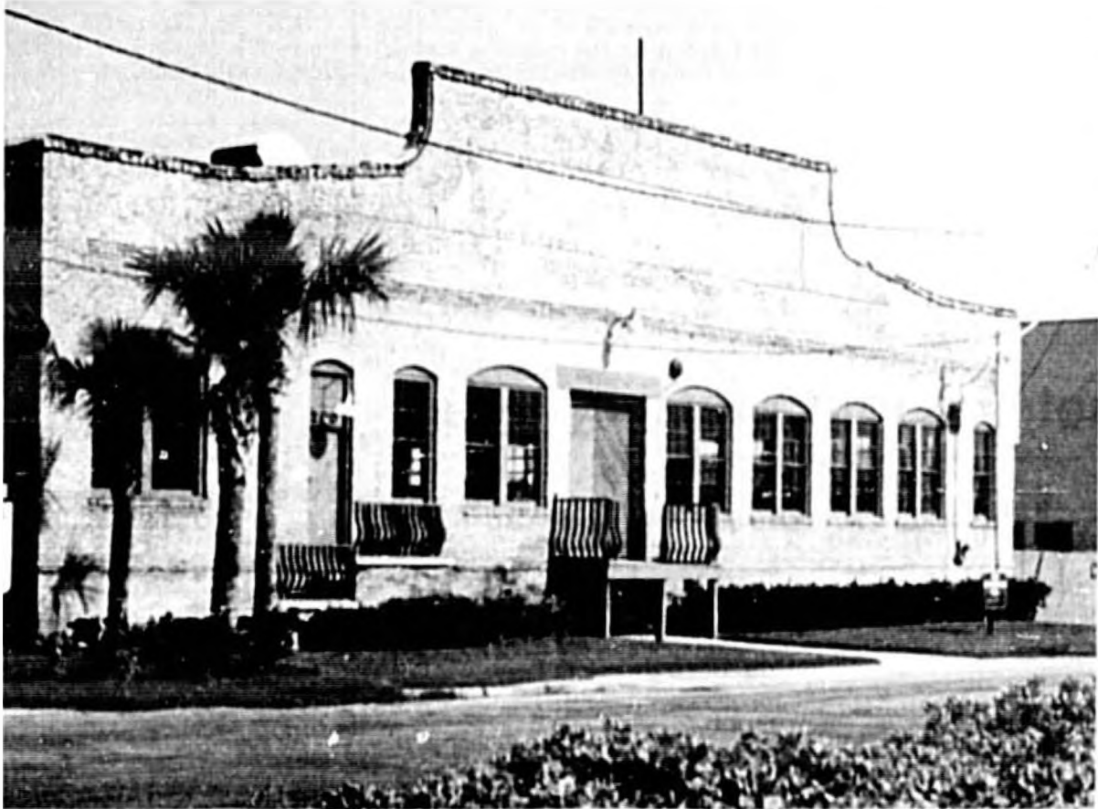
Complete Renovations, 315 E. Second St. Sanford includes Crown Square among the buildings they have renovated. Crown Square also known as the Old Southern Chemical Building won the Sanford Chamber of Commerce Beautification Award in March.
