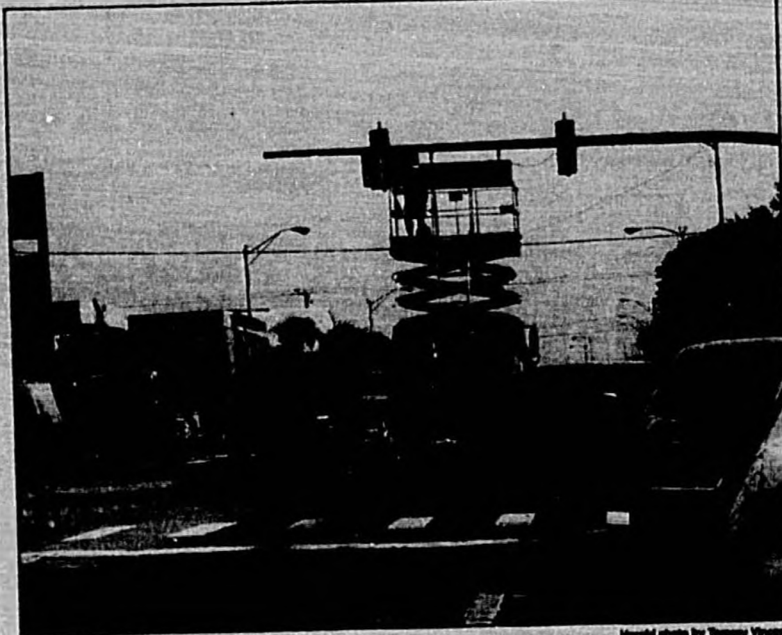
Workers from Seminole County traffic engineering finish installation of traffic signals at the intersection of U.S. Highway 17-92 and First Street, in Sanford. The new signal poles are more of an antique style than the concrete poles they replaced, but the message is still the same -- stop, go, left turn, right turn, and so on and so on and so on...
