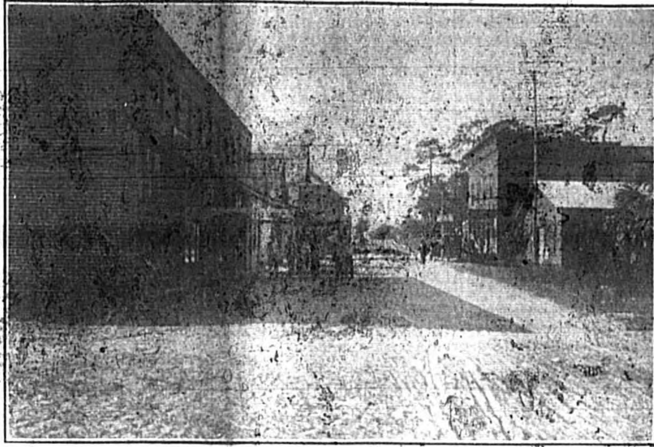
The above picture shows part of the district burned in the fire last Wednesday, in which seven entire buildings were destroyed. The brick building in the foreground is the Lawton store, and was the only building left on Main Street. Being of brick it withstood the ravages of the flames. All the buildings destroyed will be rebuilt at once, still built of brick, making a bigger and better Oviedo. The buildings on Smith Avenue are not shown in the picture.
