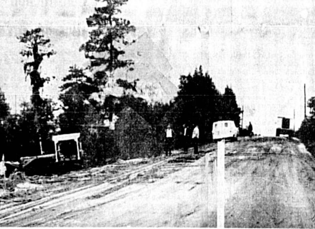
WORK BEGINS ON SAND LAKE RD. (Herald Photo)
