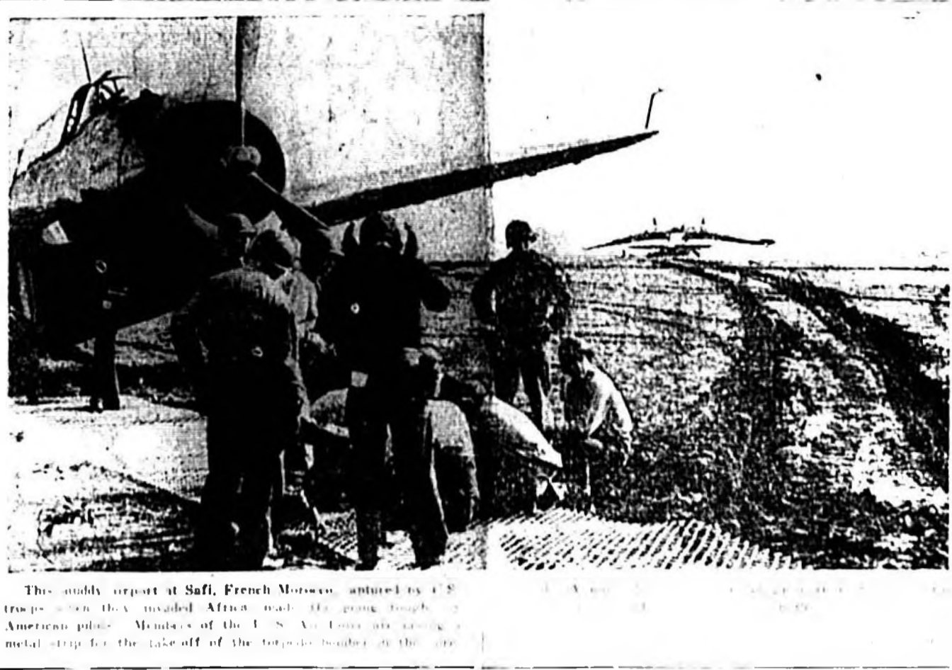
This muddy airport at Saffi, French Morocco, captured by U.S. troops when they invaded Africa, made the ground too hard for an American plane. Members of the U. S. Air Force are taking a metal strip for the take-off of the transport airplane in the foreground.
