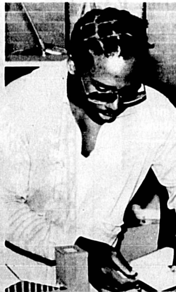
BERNARD MILLS PUTTING ON THE ROOF
