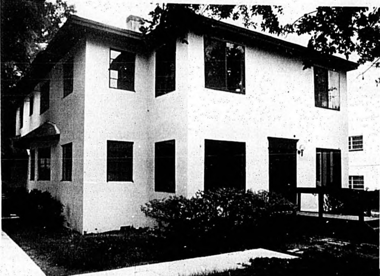
Fresh paint, a sidewalk and a ramp for wheelchairs helped give the exterior of the building a renewed image. The CITE building now has more than 5,200 square feet of usable space. The first floor houses classroom space and the low-vision
