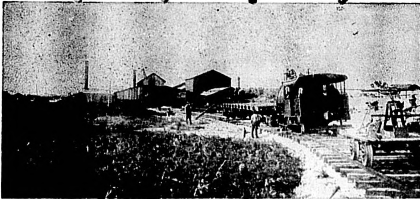
LAYING OF SECONDHAND RAILS and cross-ties began. Sands were carried to the plant, shown in background of this 1919 photo.
