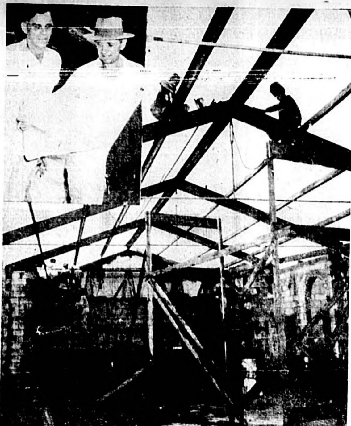
CHURCH ADDITION —Work is shown in progress on the auditorium of the new congregation of Christian Church at 21th St. and Park Ave. Shown in the inset are Ralph Lassing (left), chairman of the church building committee, and Gus Schmah, builder of the new church. Much material was salvaged from the old Congregational Church building at Third St. and Park Ave. when it was razed. The new structure is of concrete block construction and will have a stucco finish, according to Schmah, who said he looked at about 100 plans before one was decided upon. The church is being built, he pointed out, with the plan in mind of further expanding it. The church is set on a large plot, which provides plenty of space both for parking of cars and for further expansion of the building. The church when completed will be fitted with hearing aids, Schmah said, and a public address system and facilities for radio broadcasts. (Staff Photo)
