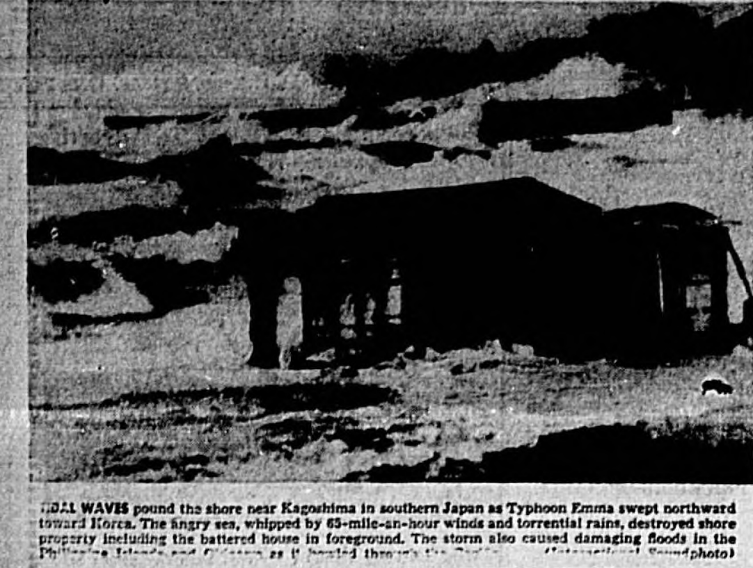
EMMA waves pelted the shore near Kagoshima in southern Japan as Typhoon Emma swept southward toward Korea. The angry sea, whipped by 45-mile-an-hour winds and torrential rains, destroyed shore property including the battered house in foreground. The storm also caused damaging floods in the Philippines and elsewhere.
