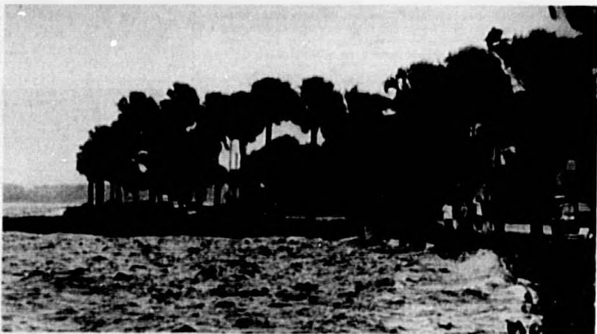
Water laps the seawall top in Lake Monroe. Officials caution passersby to watch for 'gators.'
