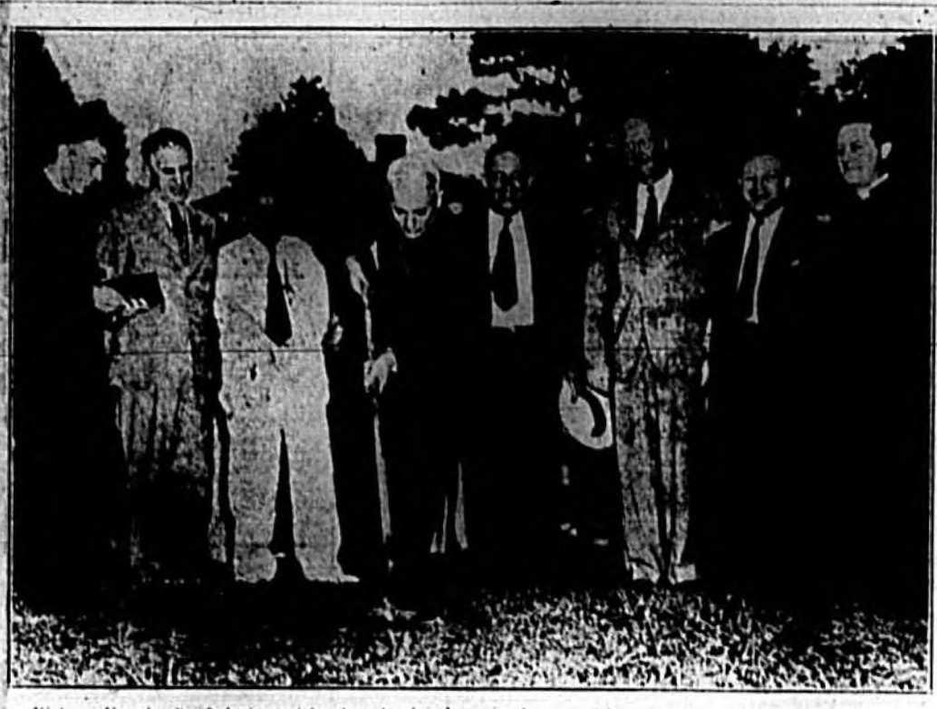
Bishop Frank A. Juhah (with shovel) is shown above taking up the first shovel full of dirt at ground-breaking ceremonies during the start of construction of the new $25,000 Episcopal student chapel at the University of Florida. Officials who participated in the ceremony are (left to right), Rev. Hamilton West, Episcopal student pastor at the University, Rudolph Weaver, director of the school of architecture and architect of the chapel, Klein Graham, representative on the building committee from the Diocese of Florida, Bishop Juhah, W. A. Shands, Gainesville, treasurer of the building committee, Dr. John J. Tiers, president of the university, Rev. Martin Bram, pastor of Holy Cross Church in Sanford and representative on the committee of the Diocese of South Florida, and Rev. Francis Wakefield, pastor of Holy Trinity Episcopal Church in Gainesville.
