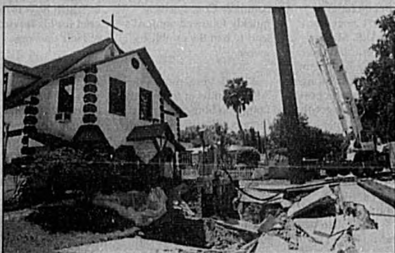
A stormwater drain collapsed in front of Victory Temple of Praise Church on Pine Avenue. The collapsed caused moderate damage to the church.
