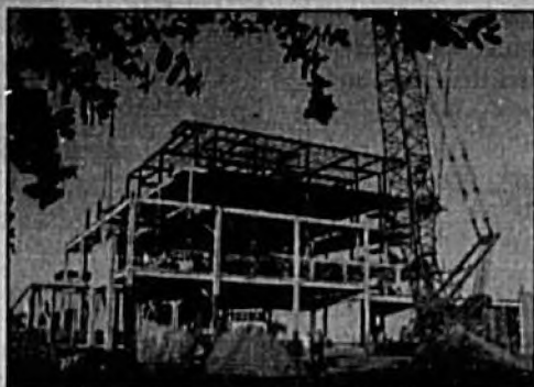
Right: Sanford's own Hardy Rawls was chosen as Of Lonely, the spokesman for Maytag appliances. Left: Significant progress was made on the construction of the new Seminole County Justice Center. Located in the Five Points area of Sanford on U.S. Highway 17/92, the new courthouse is scheduled to be finished in September 2004.
