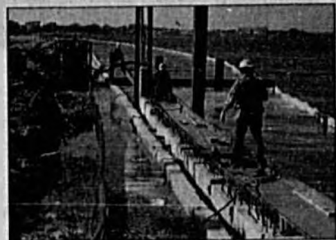
Below: Crews set some of the first seawall panels on the Sanford Riverwalk near Mellonville Avenue. Above: The final seawall panel for the Riverwalk project is installed at Memorial Park.
