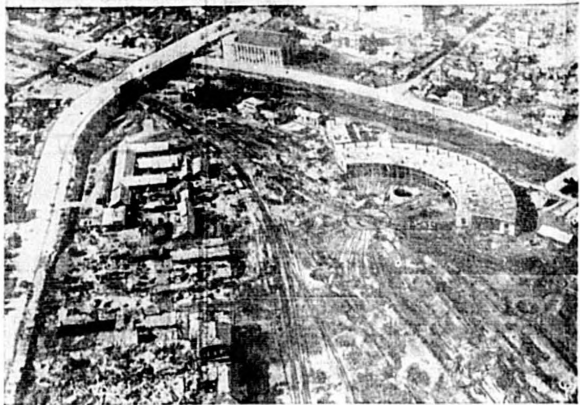
TARGET OF AMERICAN B-29 SUPERFORTRESSES, the marshaling yards and roundhouse at Watson, North Korean railroad hub, are now a mass of twisted tracks, overturned and burned-out cars and engines, and demolished buildings. The Red industrial city was recently captured.
