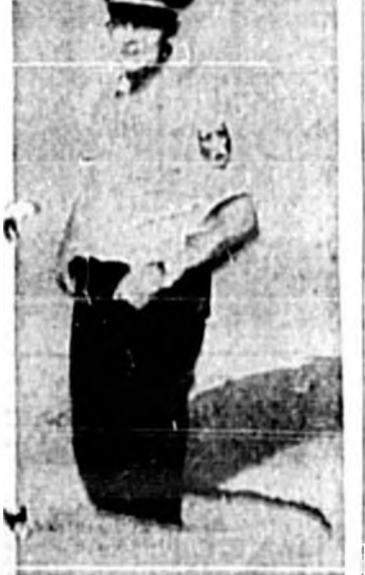
DEPUTY SHERIFF A. E. EVANS standing in a hole on East First St. at Chapman Ave. The pavement caved in apparently because the earth washed out under it during recent rains.
