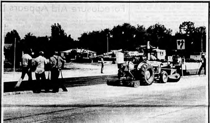
U.S. 17-92 Work Progresses
