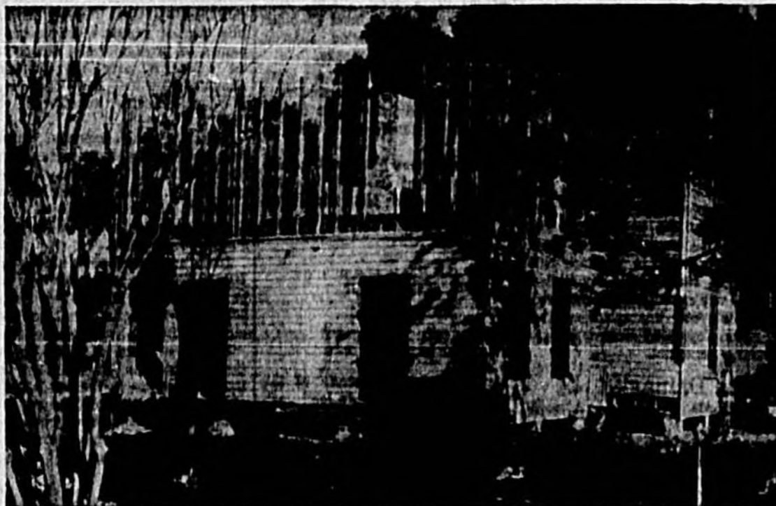
ENTERPRISE LANDMARK, known in recent years as The Dicken's Place, has been purchased by William Goodwin who plans to build a new home on the location at DeBary Ave. and Madison Pl. when wrecking of the old one is completed. (Cox Photo)
