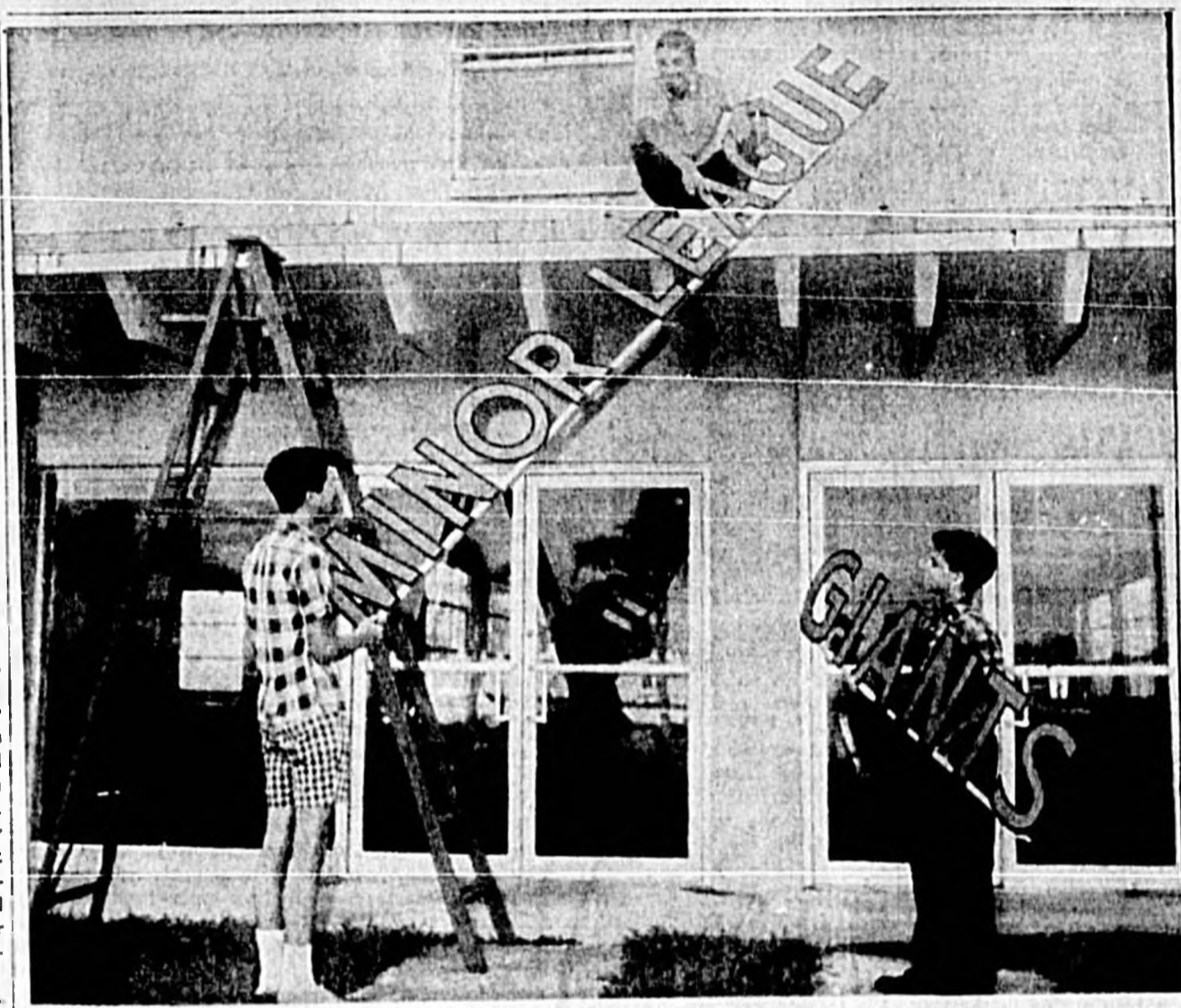
DOWN WITH THE GIANTS — ON WITH THE Cadets! Giants Minor League Training Base sign came down Thursday as work progresses on the opening of the Sanford Naval Academy, scheduled for Sept. 16. Bobby Williams (on the roof) and Johnny Williams, (holding Giants sign) sons
