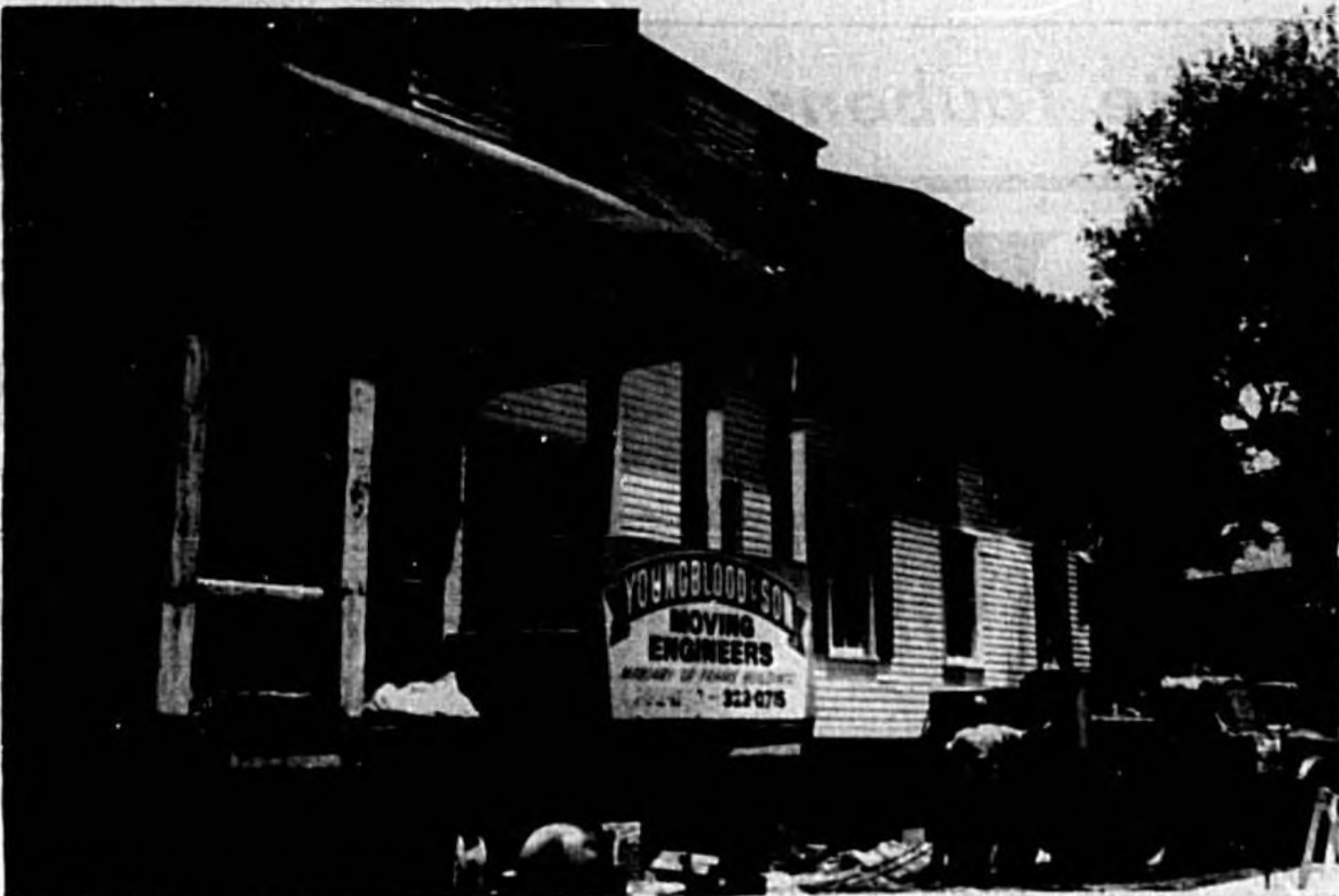
Education On The Move Rollins College is celebrating its Centennial, and the repositioning of the 100-year-old Pinehurst dormitory, plus a complete facelift for the Grande Dame, is all part of the campus improvement program. Sanford's Tommy "T.A." Youngblood & Son., house movers, uses a hydraulic jacking system to lift building.
