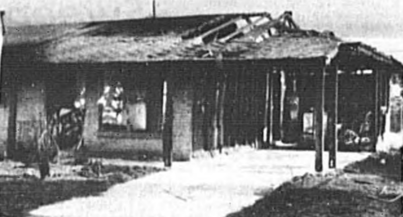
With a hole in its roof gaping skyward, the empty shell of a house is all that remains today of a home that was engulfed in flames Sunday at 162 Bethune Circle, Sanford.
