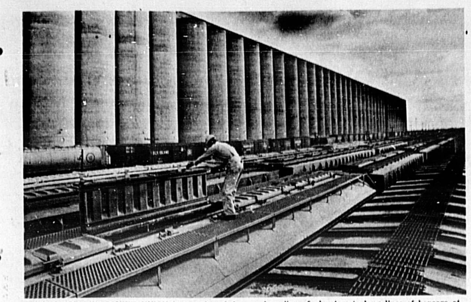
GRAIN FOR THE SOVIET UNION is transferred from a long line of elevators to long lines of boxcars at Wichita, Kans. Moving the almost half-billion bushels of wheat in the billion-dollar U.S.-Soviet deal, the largest single international grain deal in history, is pressing the nation's storage and transportation capacity.
