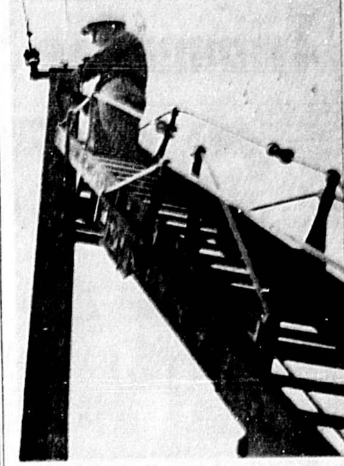
NEW STREET lights on Hwy. 17-92 from 27th St. to Onora Rd. will go into operation by Friday night. Shown above is a city workman installing one of the new lights that will "brighten up" Sanford Plaza. Some 15 lights are being installed.
