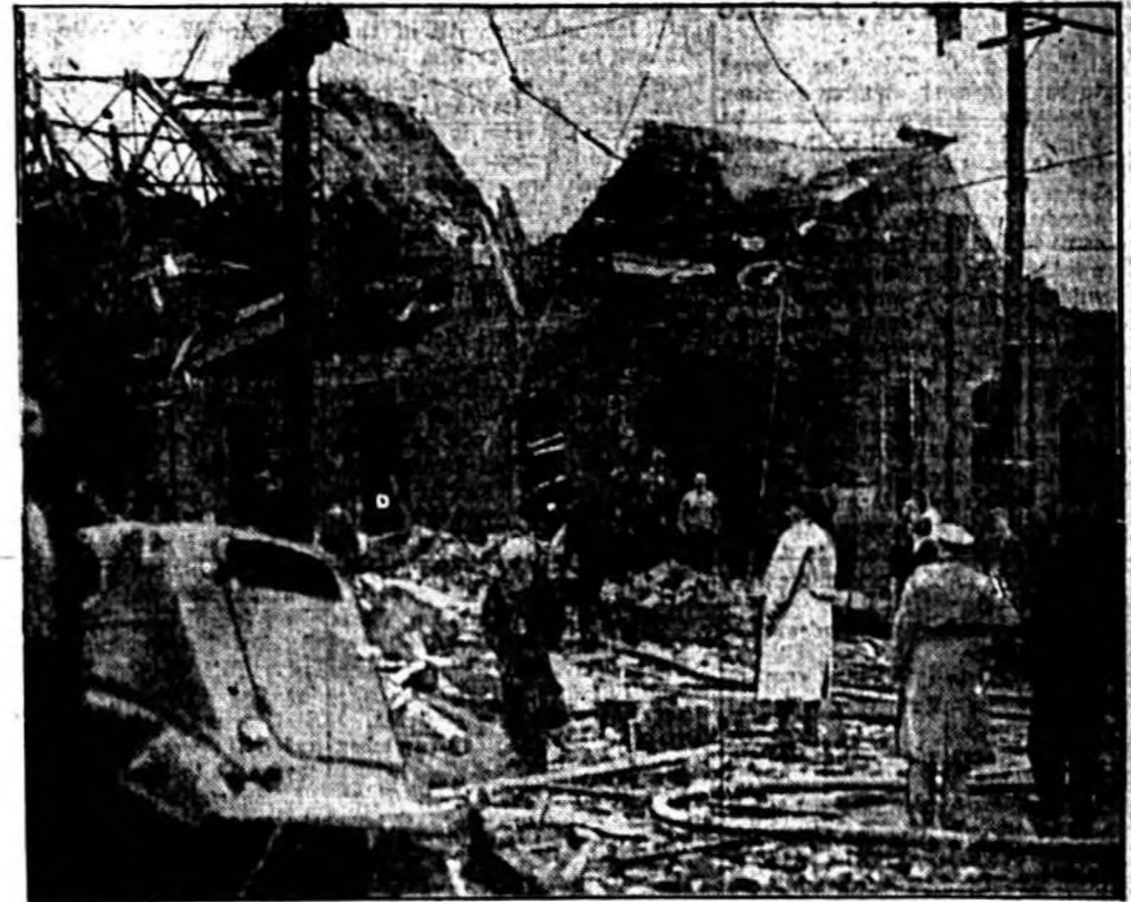
This debris was all that remained of the police station after a tornado roared through Gainesville, Ga., wrecking the business section, killing 43 persons, and injuring hundreds of others. Property damages were estimated into the millions as the twister cut a path of destruction two and a half miles long and a half mile wide through the north Georgia industrial city. (Associated Press Photo)
