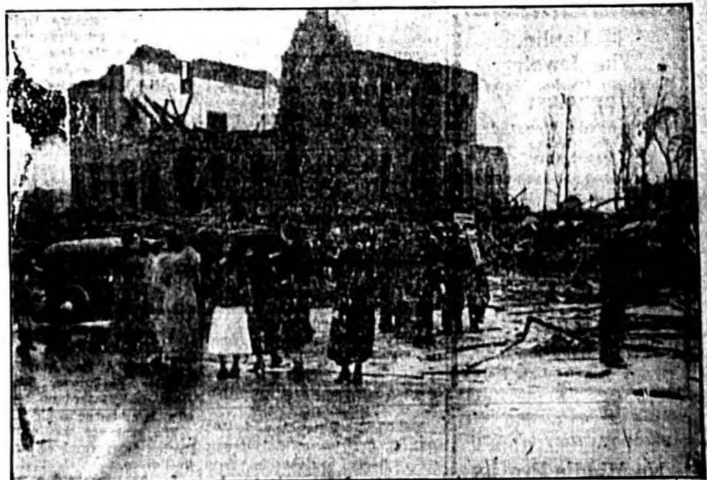
Tearing a hole through the building, a death-dealing tornado which took the lives of 43 persons caused the Gainesville, Ga., courthouse to crumble. A marble monument was the only thing left standing in the courthouse square—located in the center of the city—when the twister, followed by fire, razed the town and caused millions of dollars damages. (Associated Press Photo)
