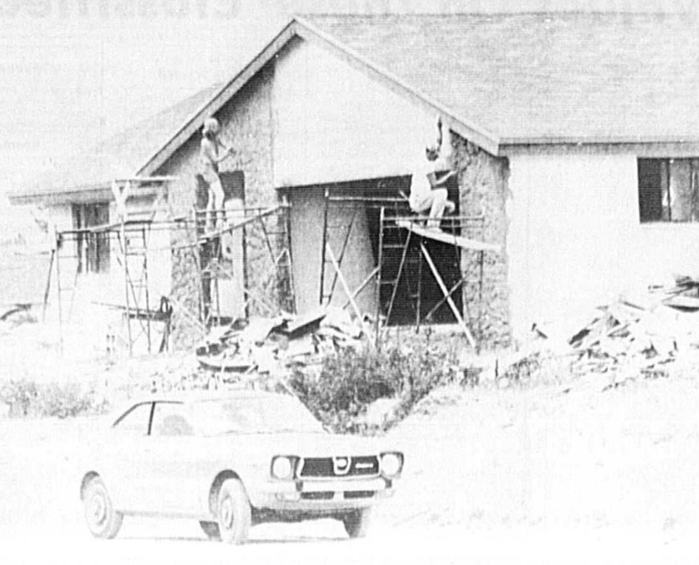
CONSTRUCTION UNDERWAY AT SKYLARK... 237 3- and 4-bedroom homes planned
