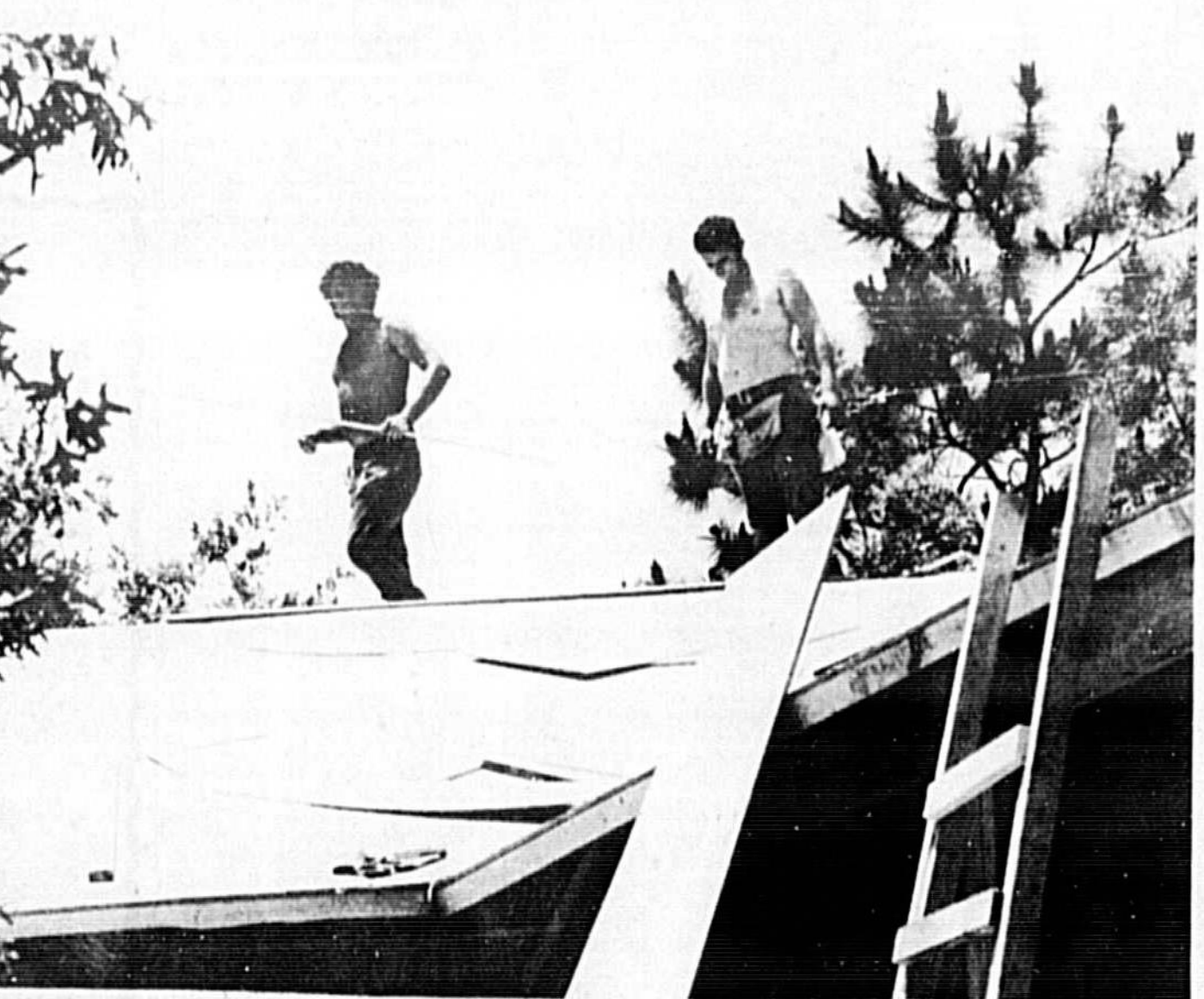
A NOTCH WAS CUT IN THE ROOF AT THIS HOUSE... To save another tree
