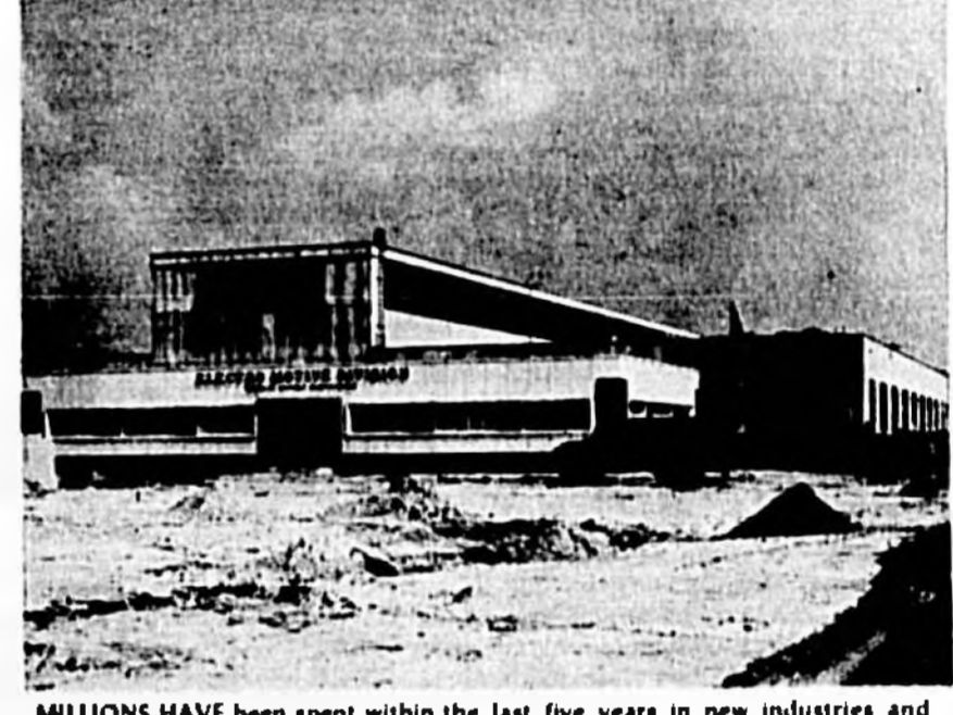
MILLIONS HAVE been spent within the last five years in new industries and business plants in the state. Typical of the new industrial buildings is this one at Jacksonville.
