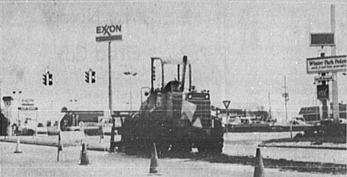
CONSTRUCTION ON U.S. 17-92-S.R. 436 INTERSECTION
