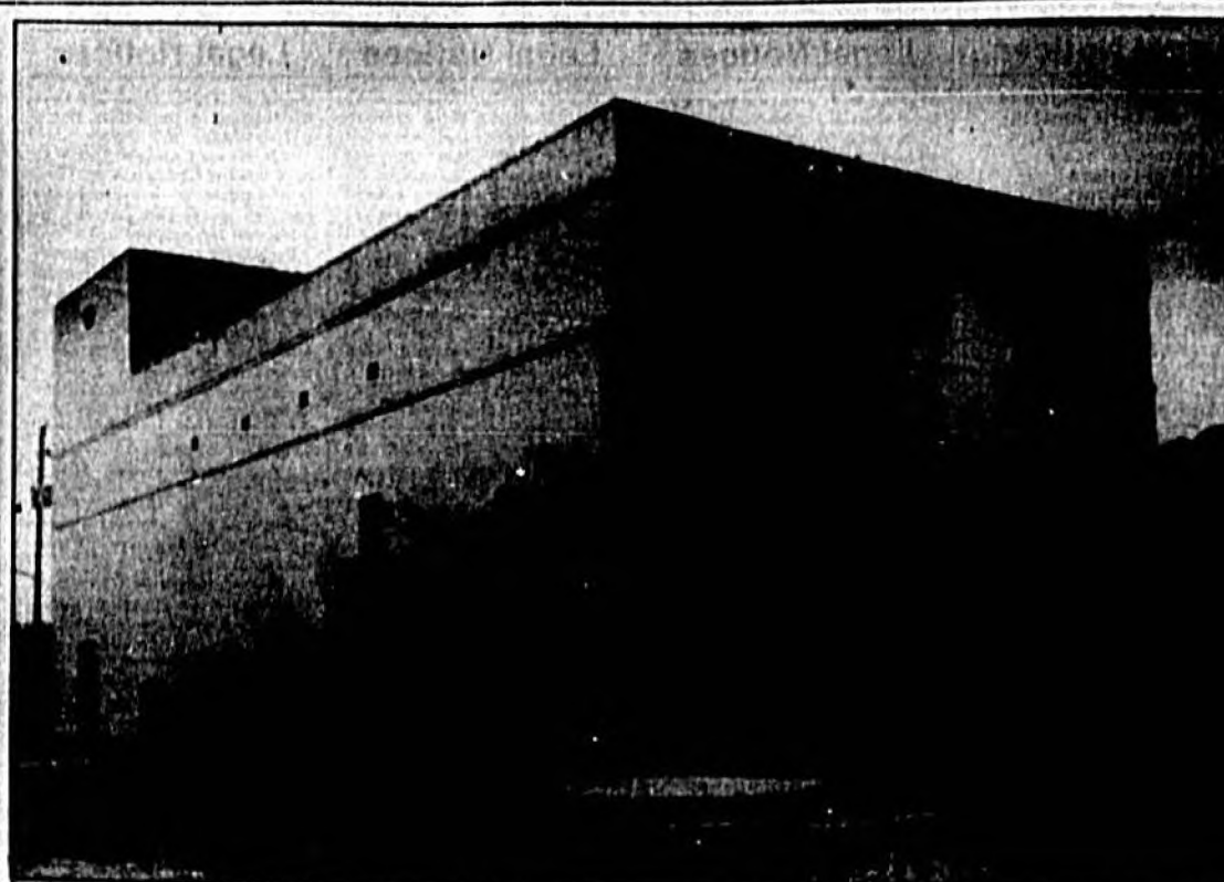
The Ritz Theater on Magnolia Avenue served as a movie theater during the 1970s. During the ongoing renovation, windows were removed for life safety issues are being stored in the building next door
